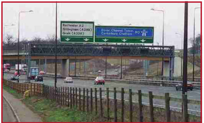
Motorway gantry signs
